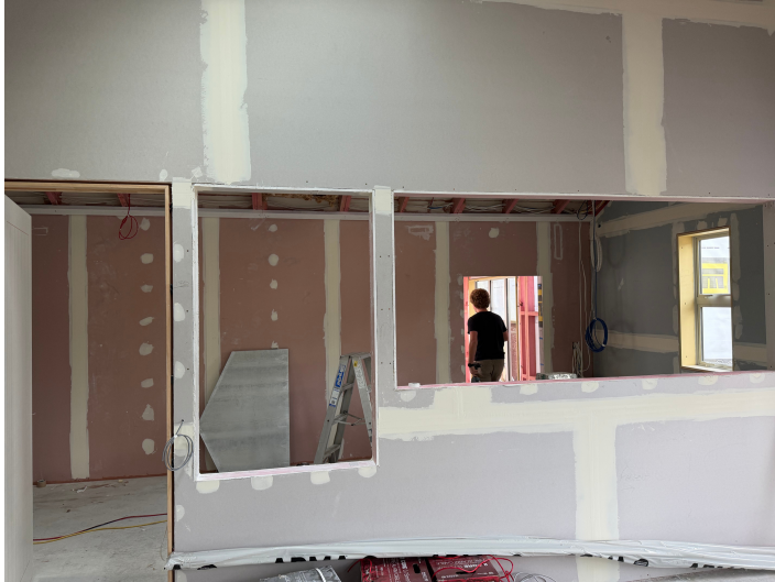
Gib stopping begins on the new reception
