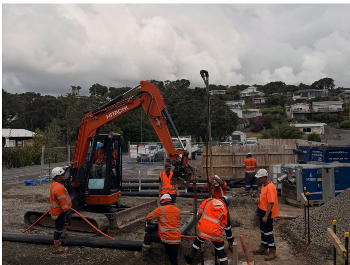
Civil works begin - Front Entrance Development
