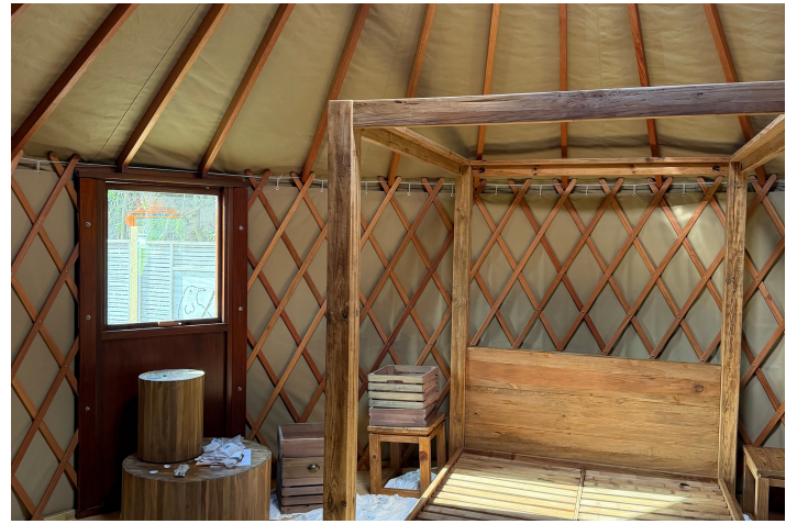
Yurt fit out work begins
