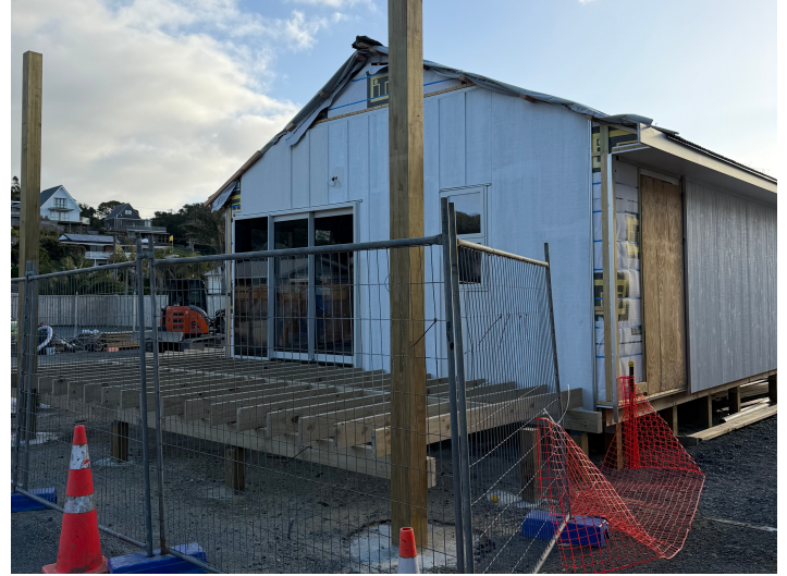
Construction new building deck commences
