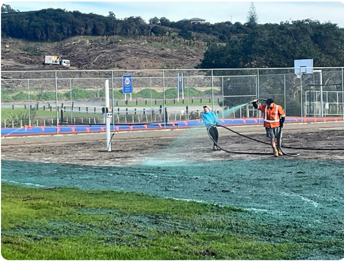
Hydroseeding Zone A and after completed site works
