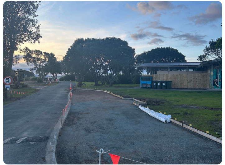
Dump station area ready for concrete to be poured
